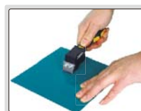
step 1: make grid cutting on surface
